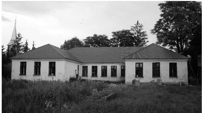
The renovated school building in Rát
